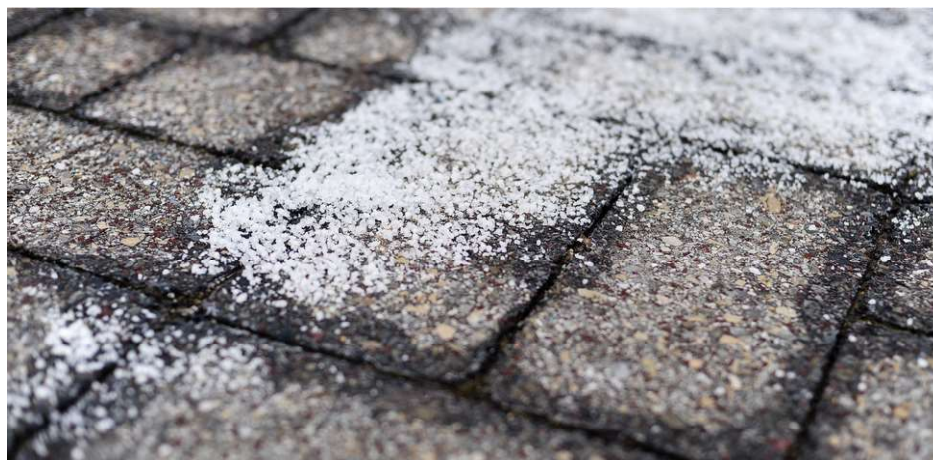
Figure 11.21 Rock salt ( NaCl ), calcium chloride ( CaCl_2 ), or a mixture of the two are used to melt ice. (credit: modification of work by Eddie Welker)
