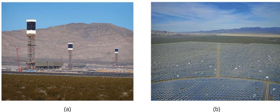
Figure 9.10 (a) The Ivanpah solar thermal plant uses 170,000 mirrors to concentrate sunlight on water-filled towers. (b) It covers 4000 acres of public land near the Mojave Desert and the California-Nevada border. (credit a: modification of work by Craig Dietrich; credit b: modification of work by “USFWS Pacific Southwest Region”/Flickr)
