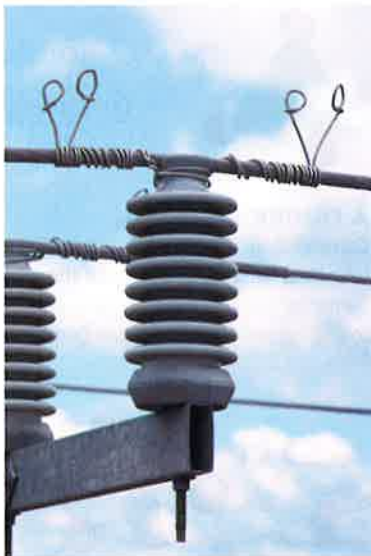
▲ Ceramic electrical insulator
